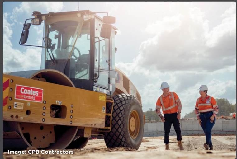
Image: Hutchinson Builders
