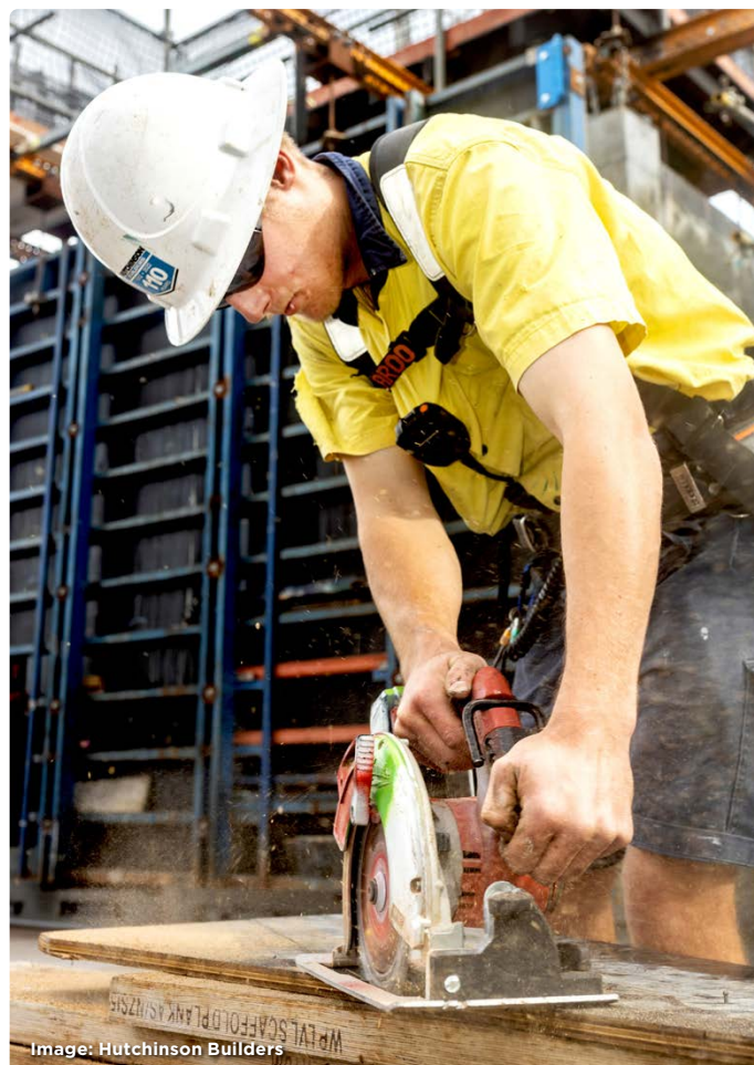
Image: Hutchinson Builders
